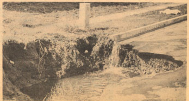
RUSHING WATER crumbles ground and streets in front of Eisenhower.
